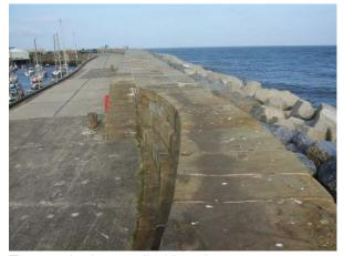
The new harbour wall with rock armour, tetrapods and raised section (Asset Ref No. 1221D901D1301C01)
