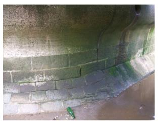
Cracking in the sea wall and footing of the Lifeboat Station (Asset Ref No. 1221D901D1301C08)
