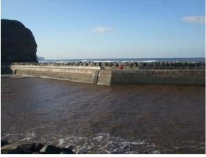
Rock armour lines the seaward side of the breakwater (Asset Ref No.1221D901D0403C03)
