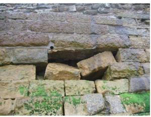
Lower section of concrete and sandstone, with blockwork wash out (Asset Ref No. 1221D901D1402C05)
