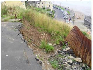
Mu28/Z recent landsliding and footpath damage (Locally Active)
