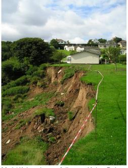
Mu24/A headscarp failure at Knipe Point
