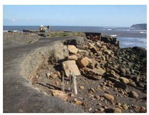
Outflanking and erosion occurring behind the breakwater
