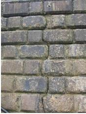
Joint cracking and loss of material from the sea wall (Asset Ref No. 1221D901D1201C07)
