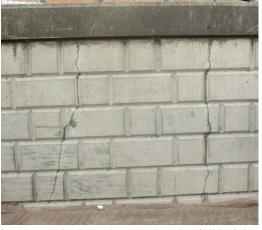
Large vertical cracks running the full height of the sea wall (Asset Ref No. 1221D901D1201C06)
