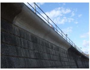
Repair work to the coping stone of the Filey sea wall
