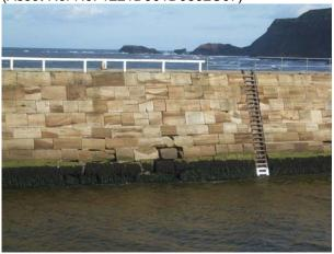
Eastern harbour arm showing mortar loss and deformation of blockwork (inspection below the water line is necessary before replacement of blocks) (Asset Ref No. 1221D901D0803C04)
