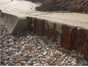
Corroded concrete and sheet pile defence at the southern end of the Sailing Club
