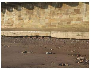
Relatively new blockwork sea wall with undercutting at the toe (Asset Ref No. 1221D901D0702C04)
