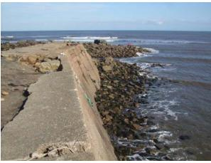
Looking along the breakwater with evidence of surface erosion (due to deformation) (Asset Ref No. 1221D901D0502C01)
