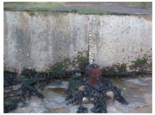
Undercutting at the toe of some parts of the harbour wall (Asset Ref No. 1221D901D0402C04)
