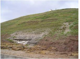
Mu11/1 degradation of slope and underlying slope stabilisation fabrics by slope wash (Inactive)
