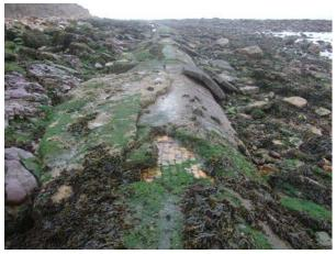
Close up of pipe at low tide showing damage to concrete surround and exposure of inner brickwork pipe (Asset Ref No. 1221D901D1201C09)
