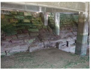
The original quay wall beneath the newer concrete jetty (Asset Ref No. 1221D901D1301C06)
