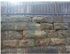
Mortar loss, surface erosion and cracking in blockwork wall (Asset Ref No. 1221D901D0802C07)
