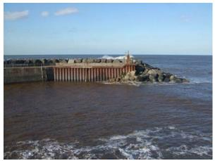
Corrosion of sheet piling on the landward side of the breakwater
