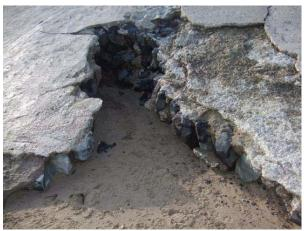
Undercutting and erosion of the concrete revetment backing Sandsend Beach (Asset Ref No. 1221D901D0702C04)
