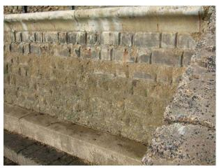
Exposed rebar and missing joints along sea wall (Asset Ref No. 1221D901D1201C03)
