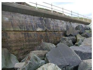
Erosion and exploitation of joints in sea wall (Asset Ref No. 1221D901D0802C03)
