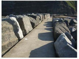
Eastern breakwater with 5-8 tonne rock armour (Asset Ref No.1221D901D0403C03)
