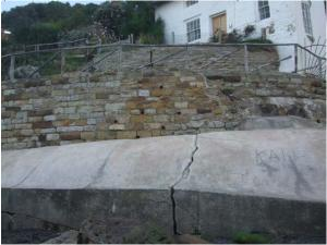
Two significant cracks propagating up through the tiered sea walls indicates active deformation (Asset Ref No. 1221D901D0601C06)
