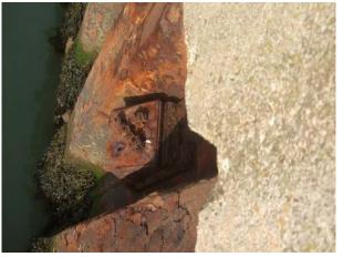
Significant corrosion of steel piling (Asset Ref No. 1221D901D1301C17)
